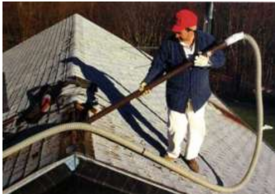
Figure 3: Installing attic insulation from the roof.
